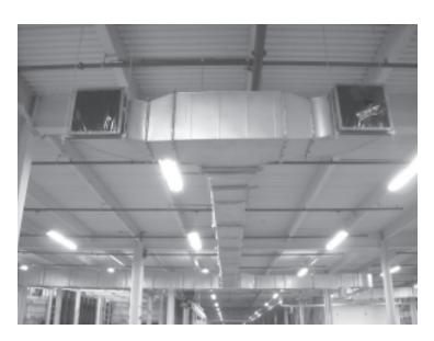
Several months back Don Park USA from Conley, Georgia and Action Electrical & Mechanical Contractors from Smyrna, Georgia teamed up to take on the fabrication and installation of duct work for the Paint Facility at the new Kia plant in West Point, Georgia. In less than 5 months 240,000 pounds of aluminized steel duct work and fittings were manufactured and delivered by Don Park USA and installed in the plant by Action Electric & Mechanical Contractors.
